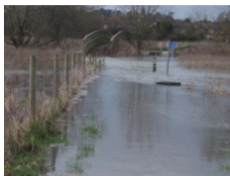
Flooding of the River Thames in north Maidenhead, 9 February 2014
